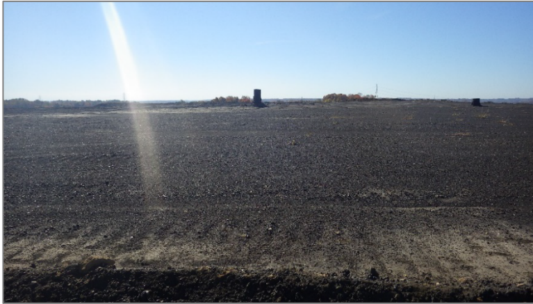
Photo 1 Phase 1 – Surface and chimney drains.
